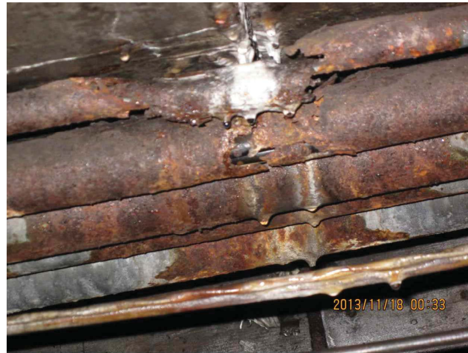
TYPICAL CONDUIT CONDITION UNDER/NEAR PLATFORM EXPANSION JOINT
